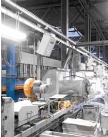
Modernisation efforts will help boost Oman Cement’s clinker production capacity.
