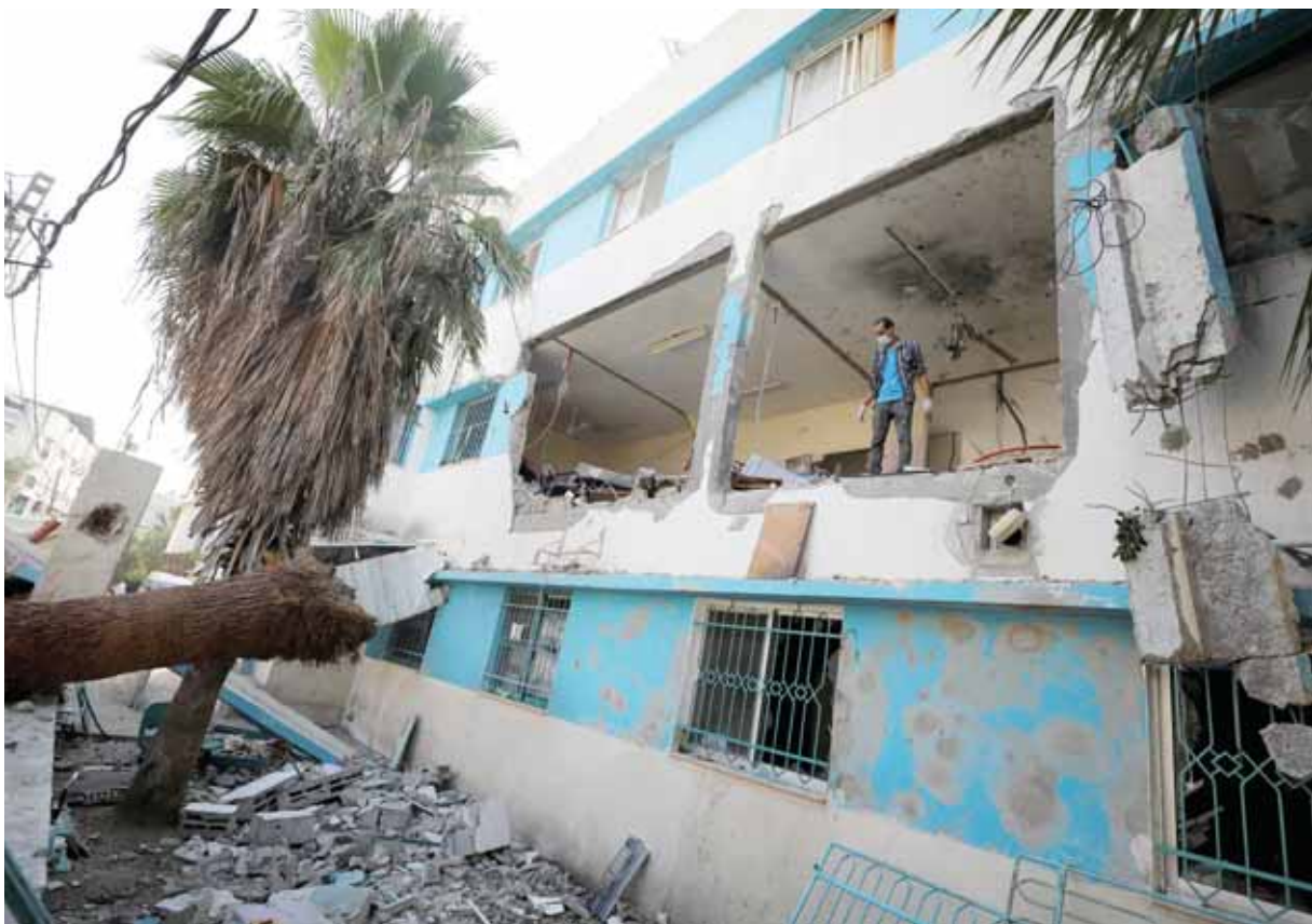
A Palestinian inspects the damages at Al Daraj clinic which was hit in an Israeli strike, in Gaza. – Reuters
