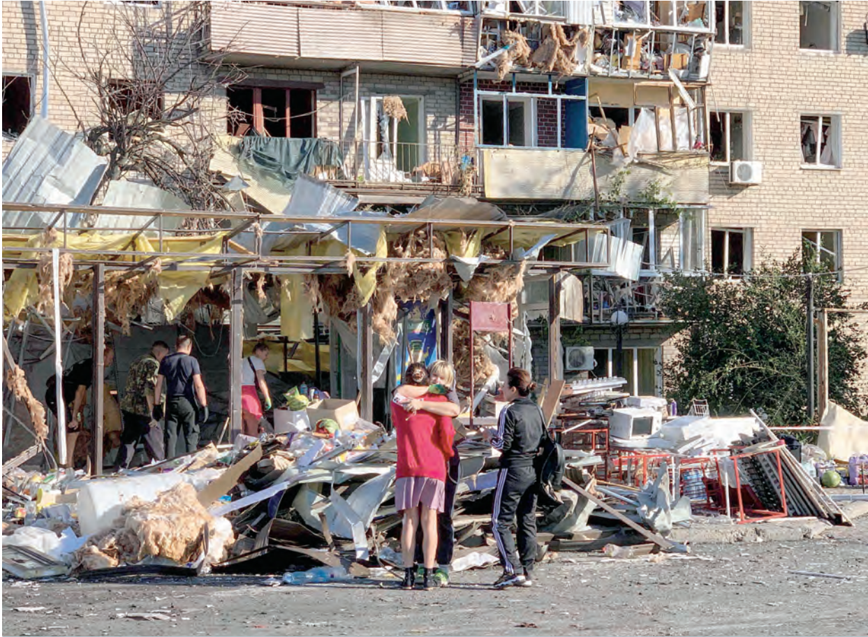
Local residents embrace each other next to a damaged residential building, in Zaporizhzhia. — AFP
