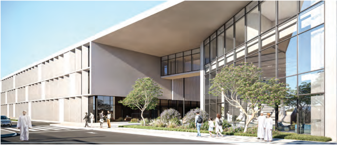
The school accommodates over 1,400 students, a modern learning environment and state-of-the-art sports facilities
