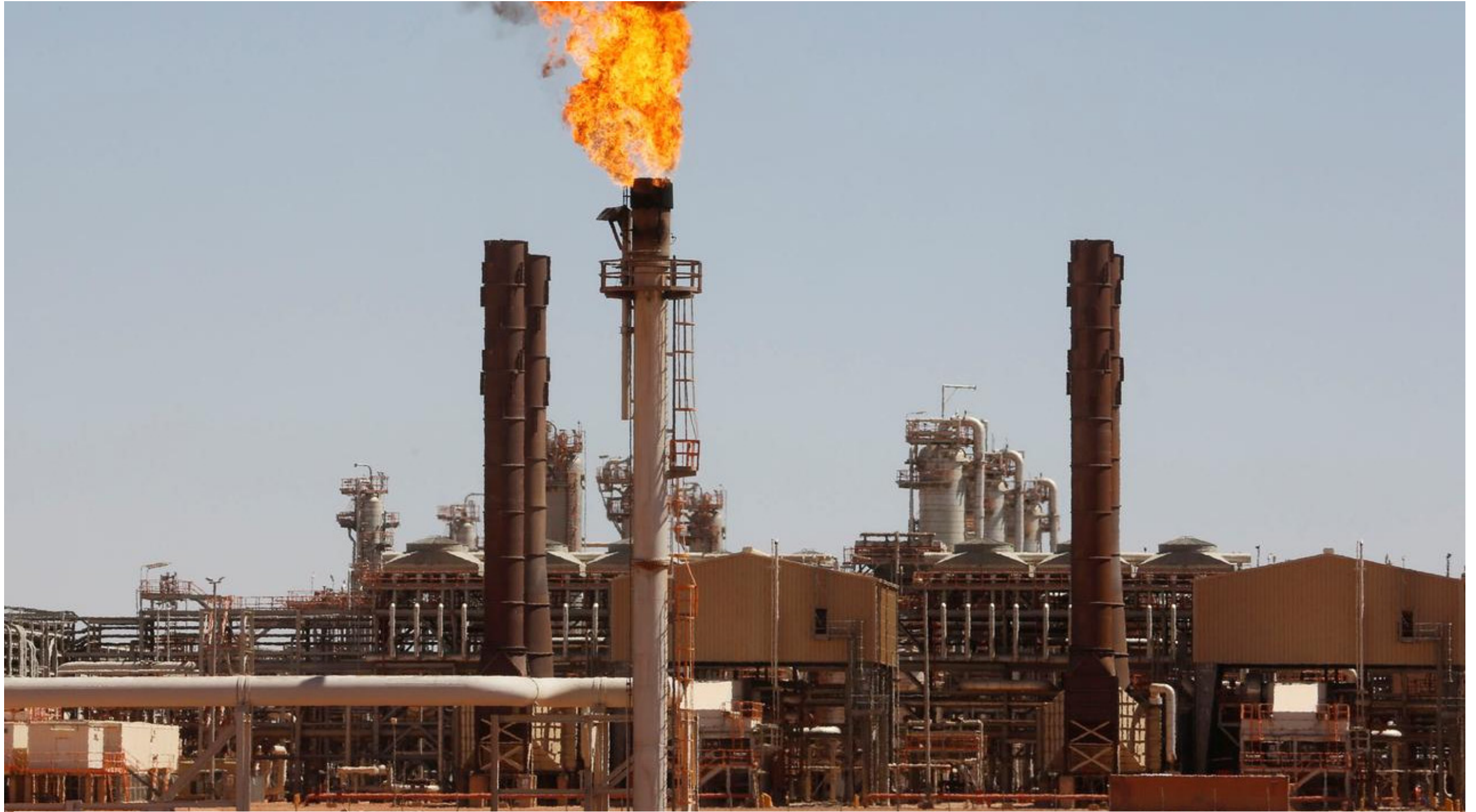
A general view of Tiguentourine Gas Plant in In Amenas, 1600 km southeast of Algiers. — Reuters
